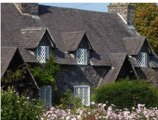
Typical Swithland slate roofed cottages.
